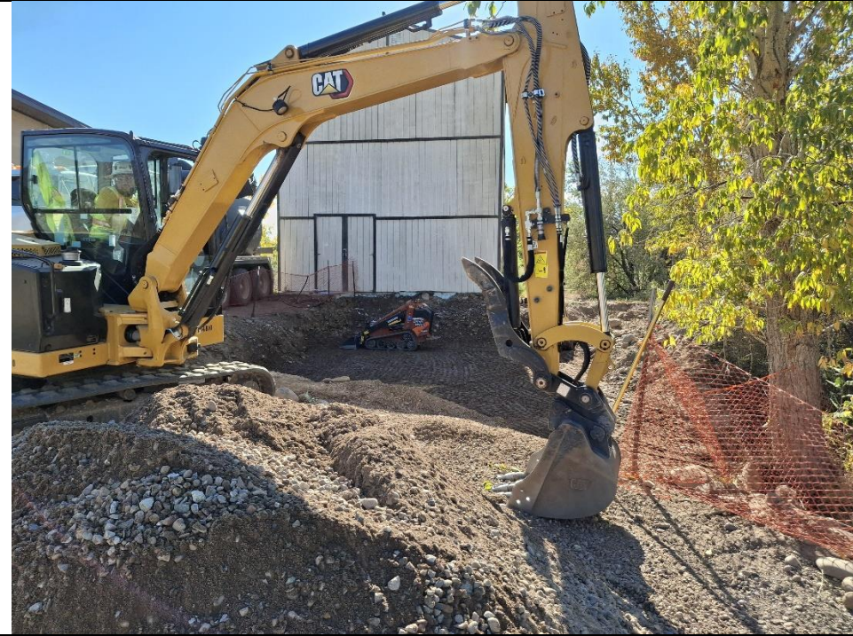
Back-up Generator Pad Excavation
